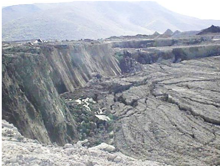
Fonte: K, Kavouridis & Agioutantis, Zach. (2006). The impact of a large-scale failure of the external waste dump to the operations at the South Field Mine, Ptolemais, Greece 10 .
